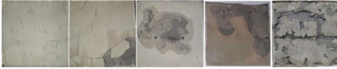
Figure 2.13: Stage 1 to Stage 5 damage of test specimens (left to right) after spalling (from Hamasaki et al. 2016)
